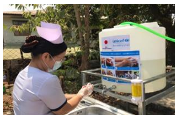
Installing hand-washing stations (UNICEF, Myanmar)
