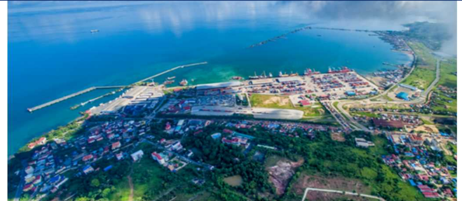
Sihanoukville Port in Cambodia (Provided by JICA)
