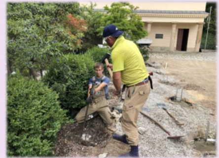
Digging a hole for making a base of prop
