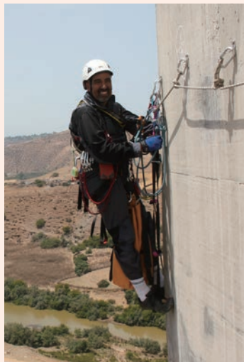
A local engineer using Ninja-Tech to carry out an inspection on a bridge of a Moroccan motorway (Photo: Tokusyu Kousyo Gijutsu Inc.)
