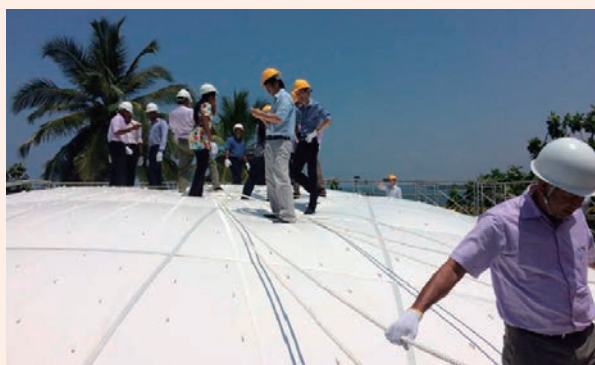
Japanese and Sri Lankan engineers checking the mounting of the Air Dome over the top of a PC Tank (Photo: ABE NIKKO KOGYO Co., Ltd.)
