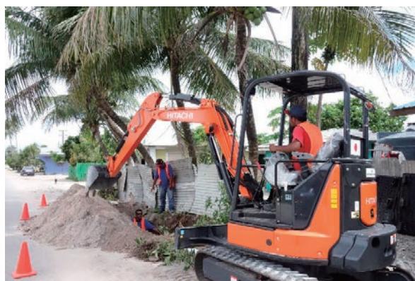
A compact excavator, procured through the Grant Assistance for Grass-Roots Human Security Project, being used to excavate soil for the installation of water pipes by the roadside in Majuro, the capital of the Marshall Islands (Photo: Chizuru Seki)
