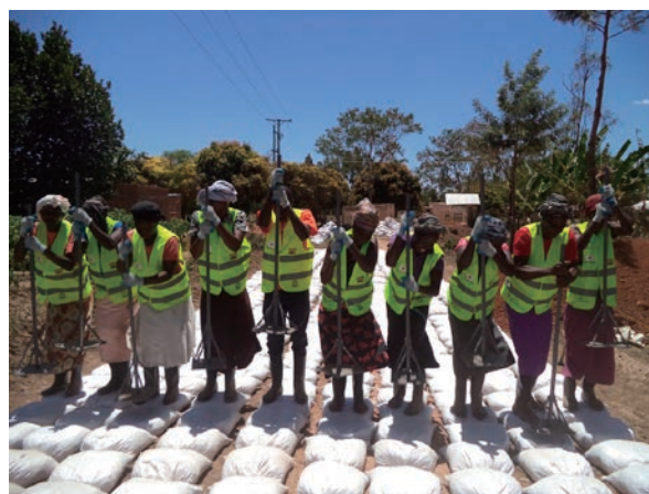
A road maintenance project being carried out using sandbags, in support of sustainable job creation and independence of youth in Kenya (Photo: NPO CORE: Community Road Empowerment)
