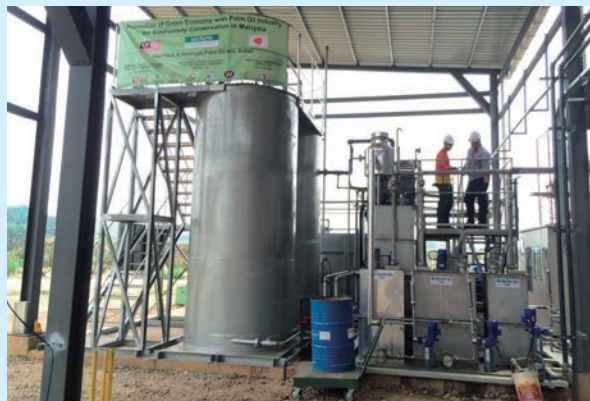
Wastewater treatment equipment, for treating palm oil wastewater and producing methane gas to be used as fuel (Photo: Professor Yoshihito Shirai, Kyushu Institute of Technology)
