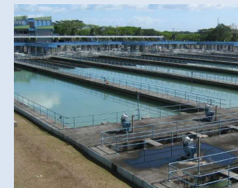
Water-related project in the Philippines (Source: JICA)
