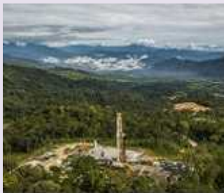
Geothermal power project in Indonesia (Source:ADB)
