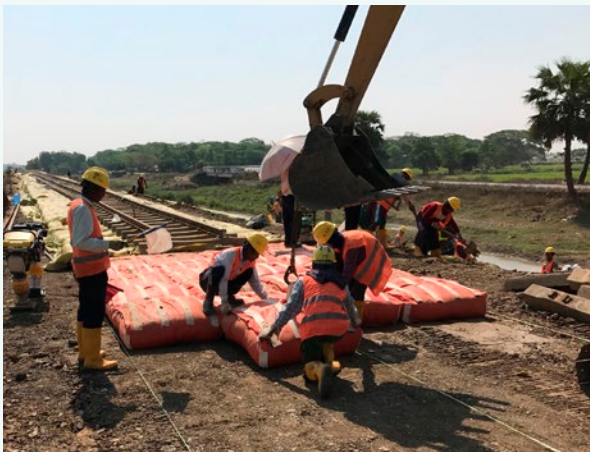
Laying D-Box sandbags for the construction of a railway line in Myanmar (Photo: Mety Co., Ltd.)
