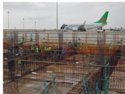
The foundation frame construction site of the international passenger terminal arrival wing (Photo: GYROS Corporation)
