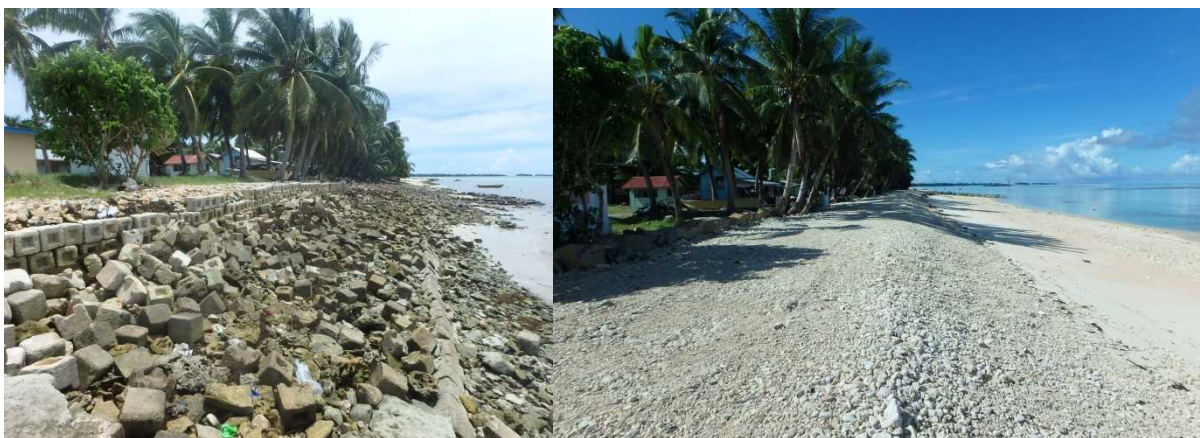
Figure 29 : Gravel nourishment at Fongafale Island of Tuvalu. Before nourishment (left) and after
