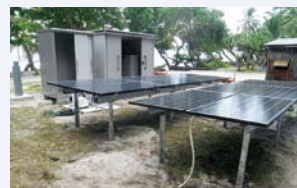
Ten solar-powered desalination plants (reverse osmosis membrane method) were installed on a remote island of Manus Province. They can desalinate sea water and purify ground water which clear the WHO drinking water standards in a location with absolutely no water or electrical infrastructure, and makes daily life possible without depending on uncertain and impure rain water. (Photo: Sojitz Corporation)
