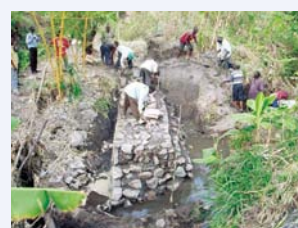
Weirs have been upgraded to masonry construction in the regions where irrigation farming with simple weirs is implemented successfully. (Photo: JICA)
