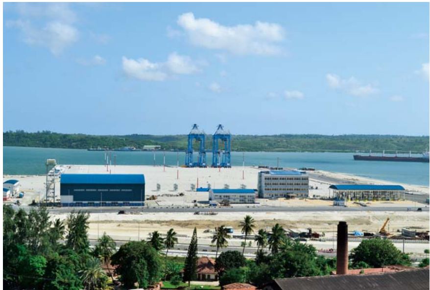
Mombasa Port, the largest commercial port in East Africa. It is the sole international trade port in Kenya, and also serves as a critical gateway port for inland countries of Africa such as Uganda and Rwanda. (Photo: Toyo Construction Co., Ltd.)
