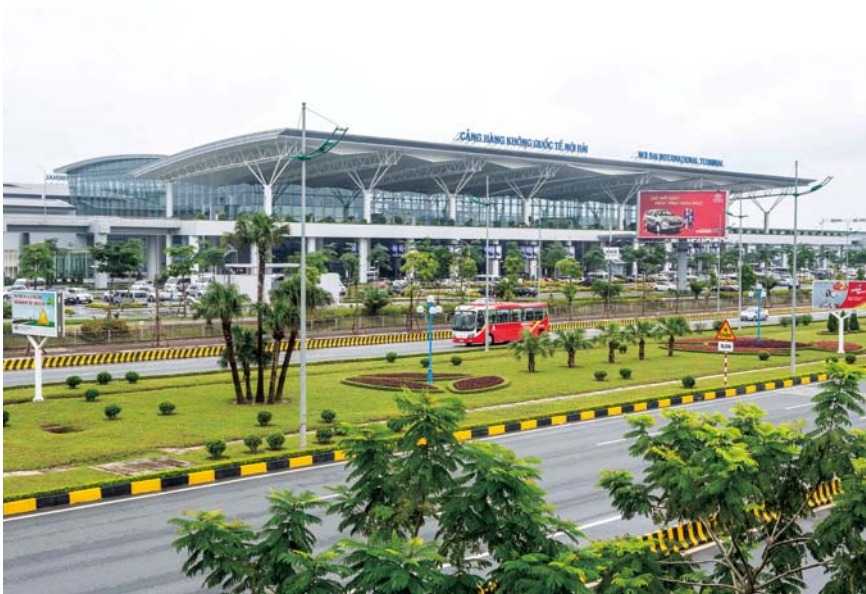
The Terminal 2 Passenger Building for international flights at Noi Bai International Airport, Viet Nam, which has large capacity for 10 million passengers (Photo: Shinichi Kuno / JICA)
