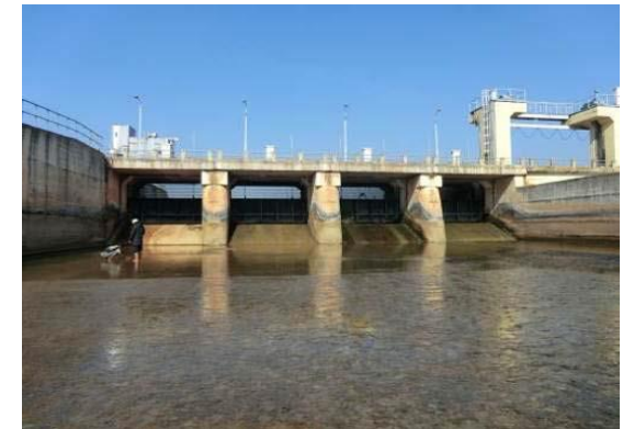
View of the plant's water intake gate
