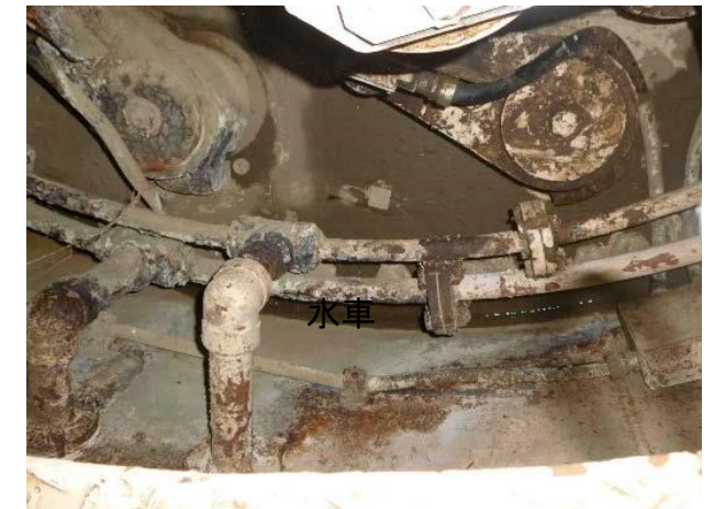
Rusted pipes
