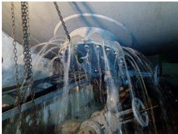
Leak from the water wheel's storage container
