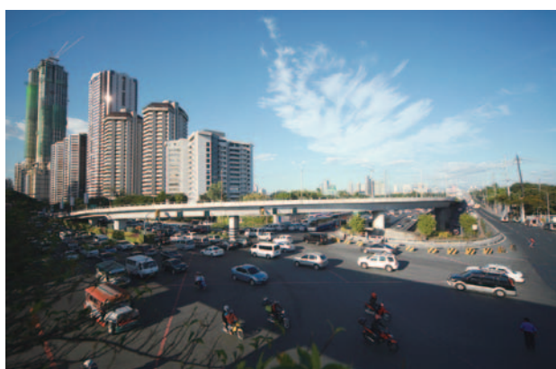
An interchange built in the business district of the City of Makati, the Philippines, as part of the Metro Manila Interchange Construction Project. The interchange contributes to alleviation of traffic congestions. (Photo: Harvey Tapan)
