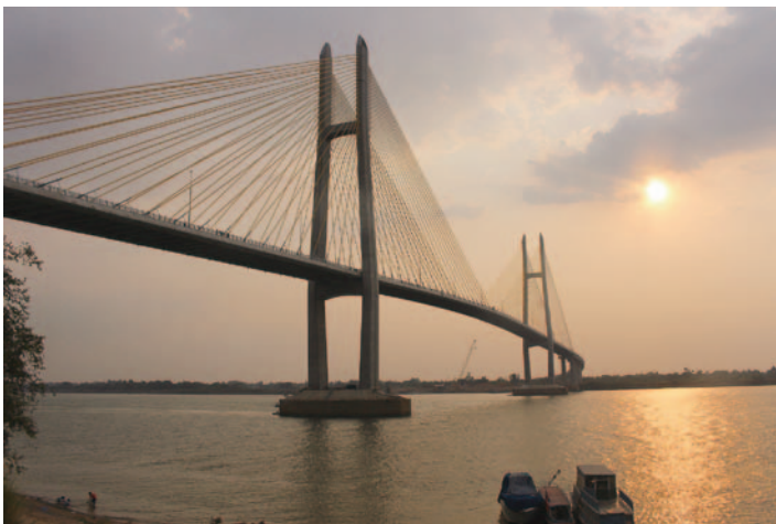
The Neak Loeung Bridge prior to its opening to traffic, after the removal of the construction cranes. The bridge was named Tsubasa Bridge because it looks like two birds spreading their wings (tsubasa in Japanese). (Photo: Shinichi Kuno / JICA)
