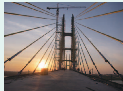
The Tsubasa Bridge. (Photo: JICA)
