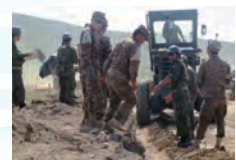
Explaining the procedure of ditch digging
