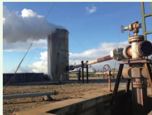
Testing steam discharge for the Guanacaste Geothermal Development Sector Loan - Las Pailas II. (Photo: JICA)
