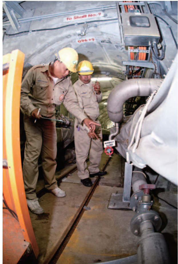
Underground transmission cables that connect Chidlom and Bangkapi substations in central Bangkok, Thailand. The existing cables were damaged or deteriorated considerably, and it was difficult to maintain them. Japan provided support for the construction of the underground tunnel for transmission and the installation of two new transmission cables between the two substations. (Photo: Shinichi Kuno / JICA)
