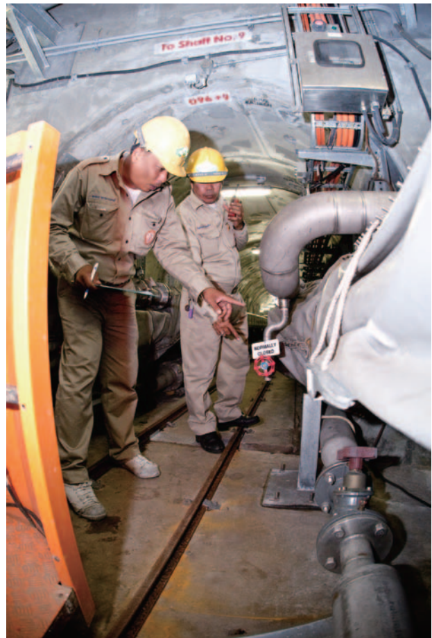
Underground transmission cables that connect Chidlom and Bangkok substation in central Bangkok, Thailand. The existing cables were damaged or deteriorated considerably, and it was difficult to maintain them. Japan provided support for the construction of the underground tunnel for transmission and the installation of two new transmission cables between the two substations. (Photo: Shinichi Kuno / JICA)
