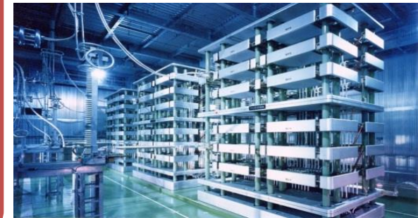
Kii Channel HVDC converter
