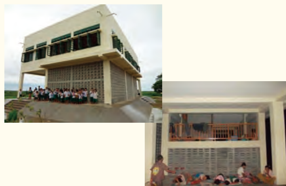
(Construction of Primary School cum Cyclone Shelter in the Area Affected by Cyclone "Nargis")
