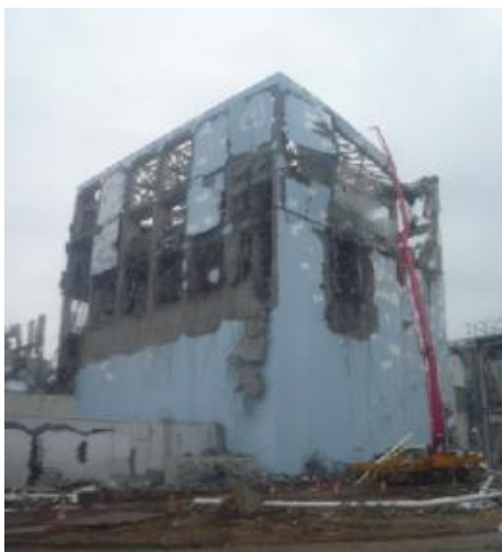
Water Injection by Concrete Pumper (3/22/2011)
