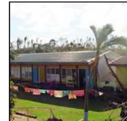
A JICA building at the school site was not greatly affected.
