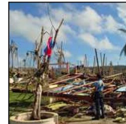
An elementary school on Samar Island, whose building was totally destroyed by windstorms
