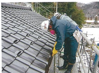
▲ Decontamination of sediment
