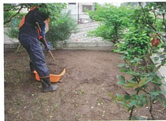
▲ Decontamination of topsoil
