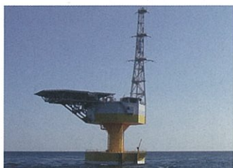
▲ Floating Offshore Substation “Fukushima Kizuna”
