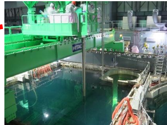
Fuel Removal from SFP (11/18/2013)
