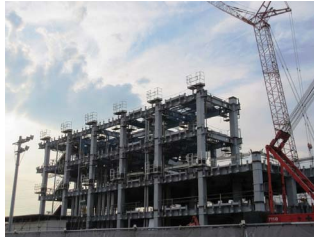
● Large rest house (under construction)
