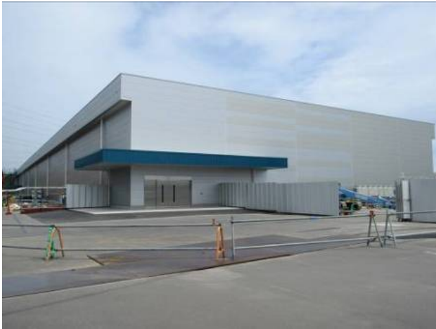
● New administration building (in operation)
