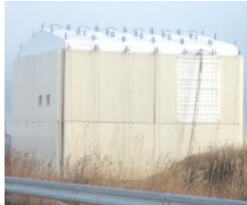
Reactor Building Cover (installed in Oct. 2011)
