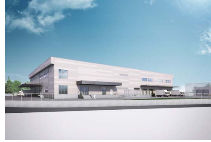
● Fukushima meal service center (under construction) OkumaTown outside the site
