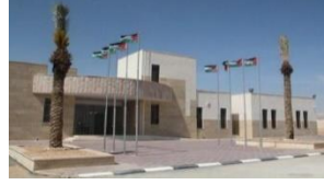
JAIP Administrative Building
