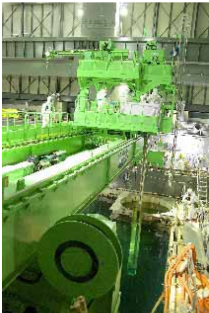
Fuel Removal from SFP
