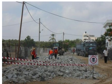
Clearance of UXOS and Rubble Removal
