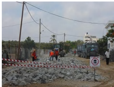
Clearance of UXOS and Rubble Removal
