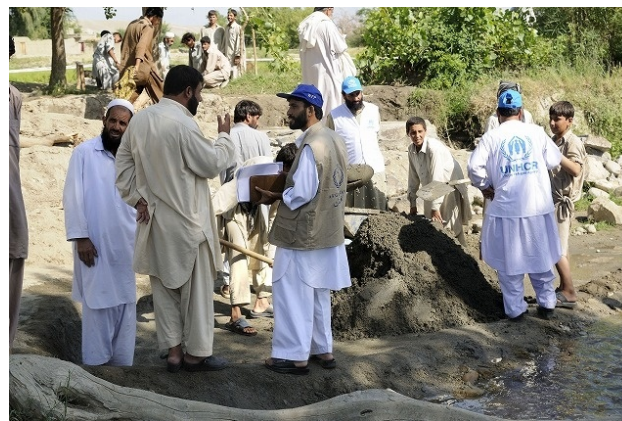
Construction of an irrigation system
