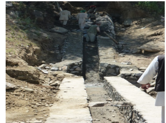
Local community improving an irrigation system under the assistance of FAO
