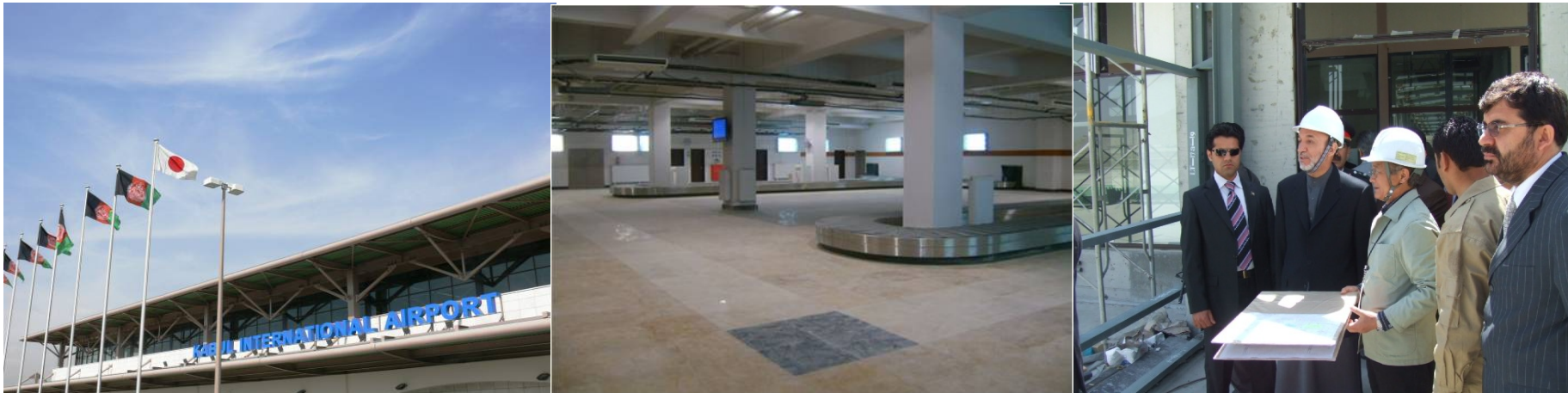
Kabul International Airport Terminal constructed with Japan's aid (President Karzai inspecting the facility)
