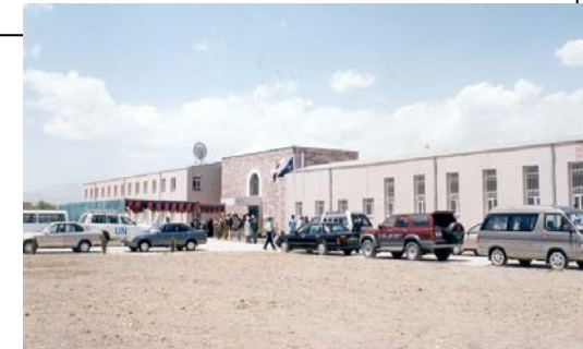
Anti-Tuberculosis Center constructed with Japan's assistance
