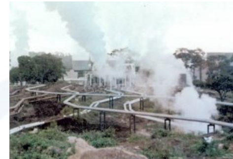
Pipeline in Ahuachapán
