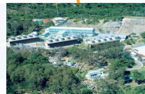
Generation Plant in Ahuachapán
