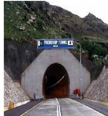
(Kohat tunnel, Northern part of the Indus Highway)
