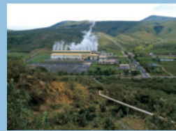
Olkaria Geothermal Power Station
