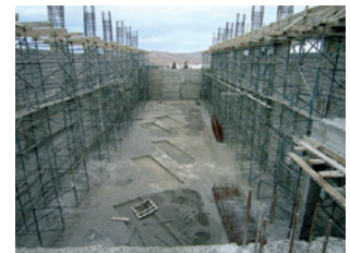
Water pumping facilities
