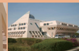
National Mubarak City Institute which will be a temporary school building (Photos: JICA)
