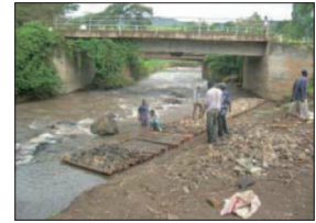
Construction of bank protection works
