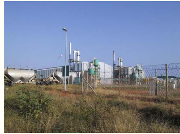
MOZAL aluminium refinement factory ( Mozambique ) A successful case of investment in Africa. The Japan Bank for International Cooperation (JBIC), the Nippon Export and Investment Insurance (NEXI) and a Japanese trade company have jointly participated in this project.
