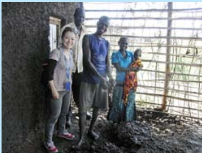
The shelter project for returnees in Central Equatoria State
