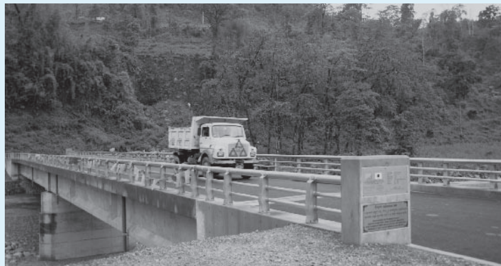
A replaced bridge that has increased resistance to natural disaster (Photo: JICA)
