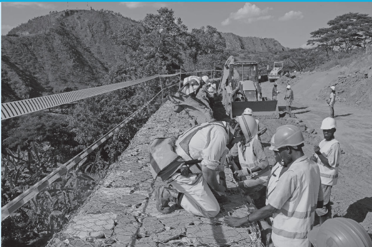
A Japanese engineer working and giving guidance at the Rusumo International Bridge that connects Tanzania and Rwanda (Photo: Takeshi Kuno / JICA)
