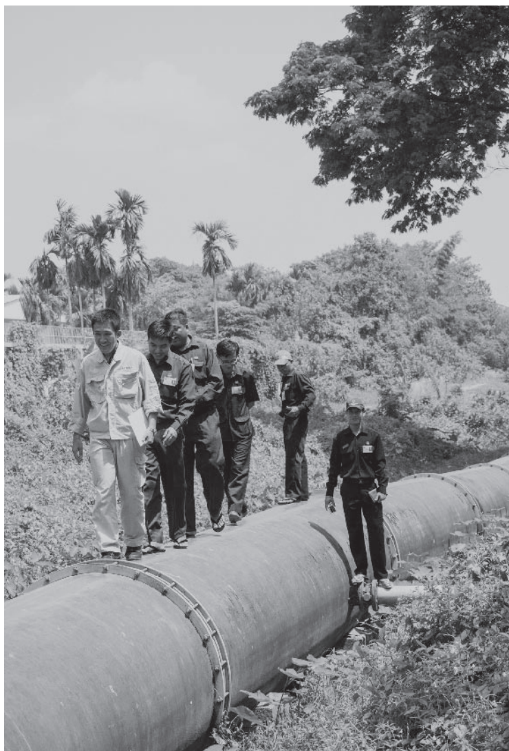
A JICA expert, Mr. Matsuoka, from the Fukuoka City Waterworks Bureau and Yangon City staff in charge of water supply inspecting the current state. (Photo: Mika Tanimoto / JICA)
