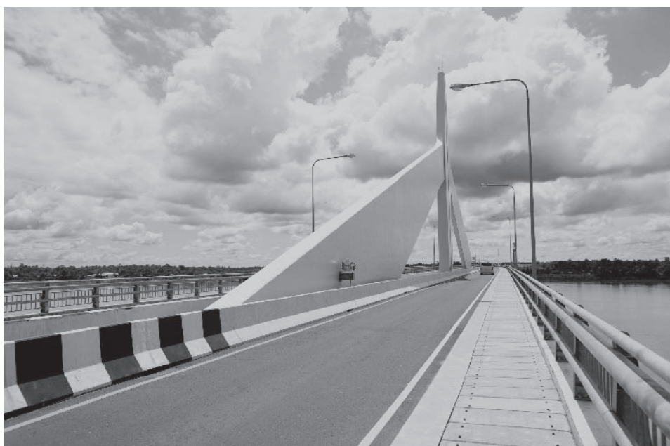
The Second Mekong International Bridge, constructed through an ODA Loan (Second Mekong International Bridge Construction Project), connects Thailand and Laos, spanning a distance of approximately 1,600 m (Photo: Yasuhiko Okuno / JICA)
