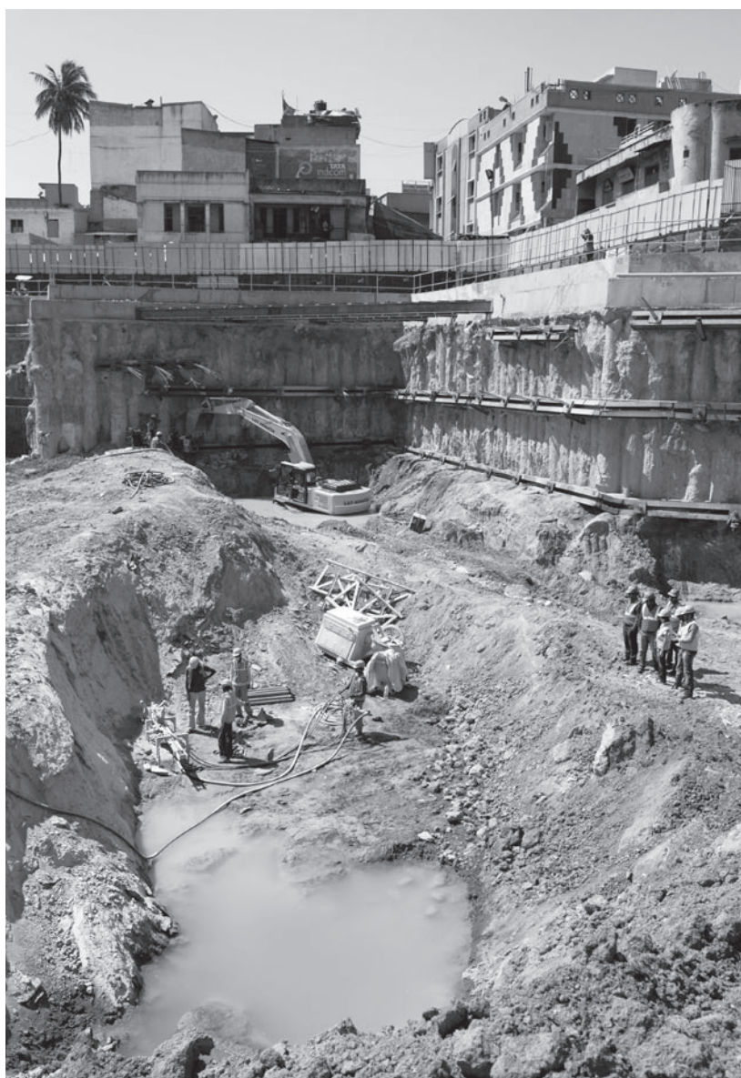
Construction site of metro in Bangalore, India. Excavation work at the Chickpete Station, where the density of building is high. (Photo: Shuhei Fujita)
