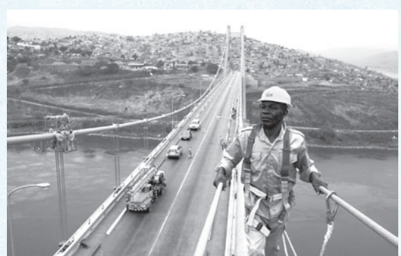
OEBK workers maintain Matadi Bridge (Photo: Shinichi Kuno / JICA)
