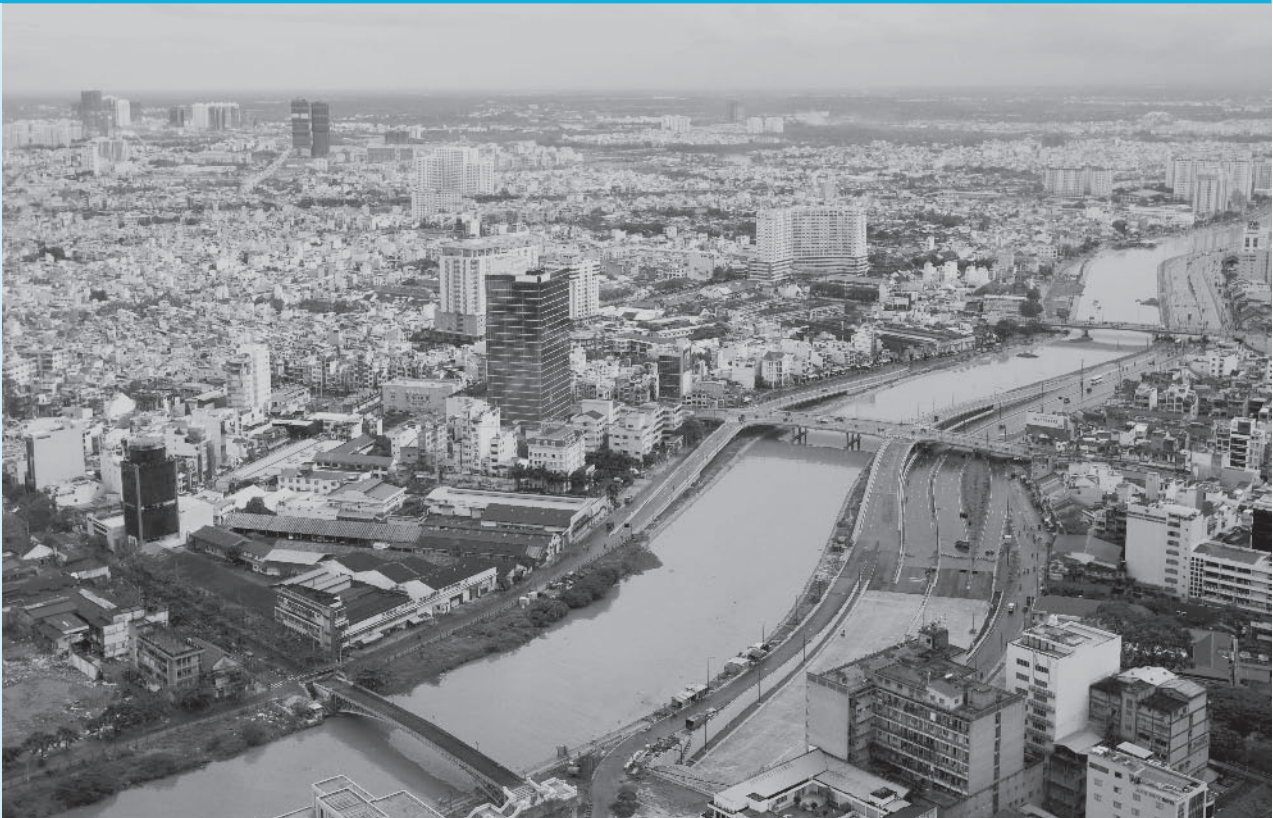
Ho Chi Minh City overlooking the Saigon East-West highway tunnel under construction in Viet Nam (Photo: Hikaru Nagatake / JICA)
