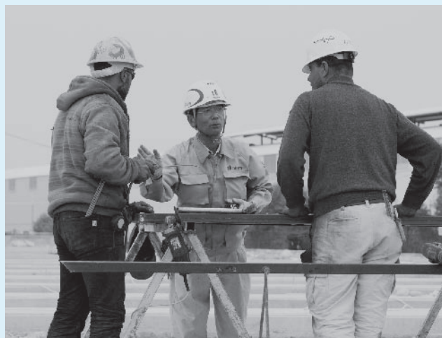
A lead member of the Japanese subcontractor at the site giving guidance to local workers (Photo: Shinichi Kuno / JICA)
