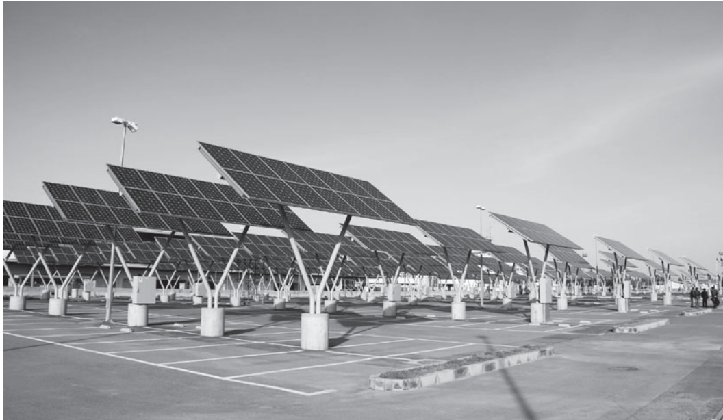
A grid-connected photovoltaic power generation system was installed at the Kabul International Airport facility in Afghanistan. Approximately 35% of electricity demand of the international terminals is provided by this system. (Photo: Sayad Jan Sabawoon / JICA)
