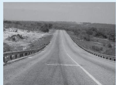
Overlooking the Nacala-Nampula trunk road (Photo: JICA)
