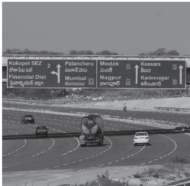
Hyderabad Outer Ring Road in India (Photo: Osamu Funao / JICA)
