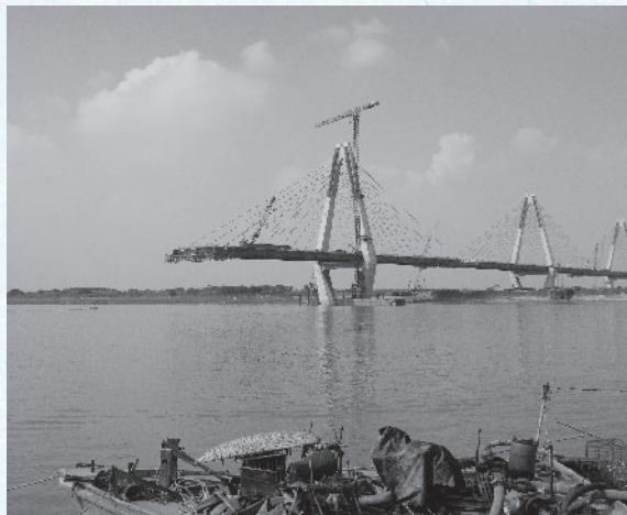
The view of the Nhat Tan Bridge during its construction from downstream of the Red River. (Photo: Yusuke Kajimura)
