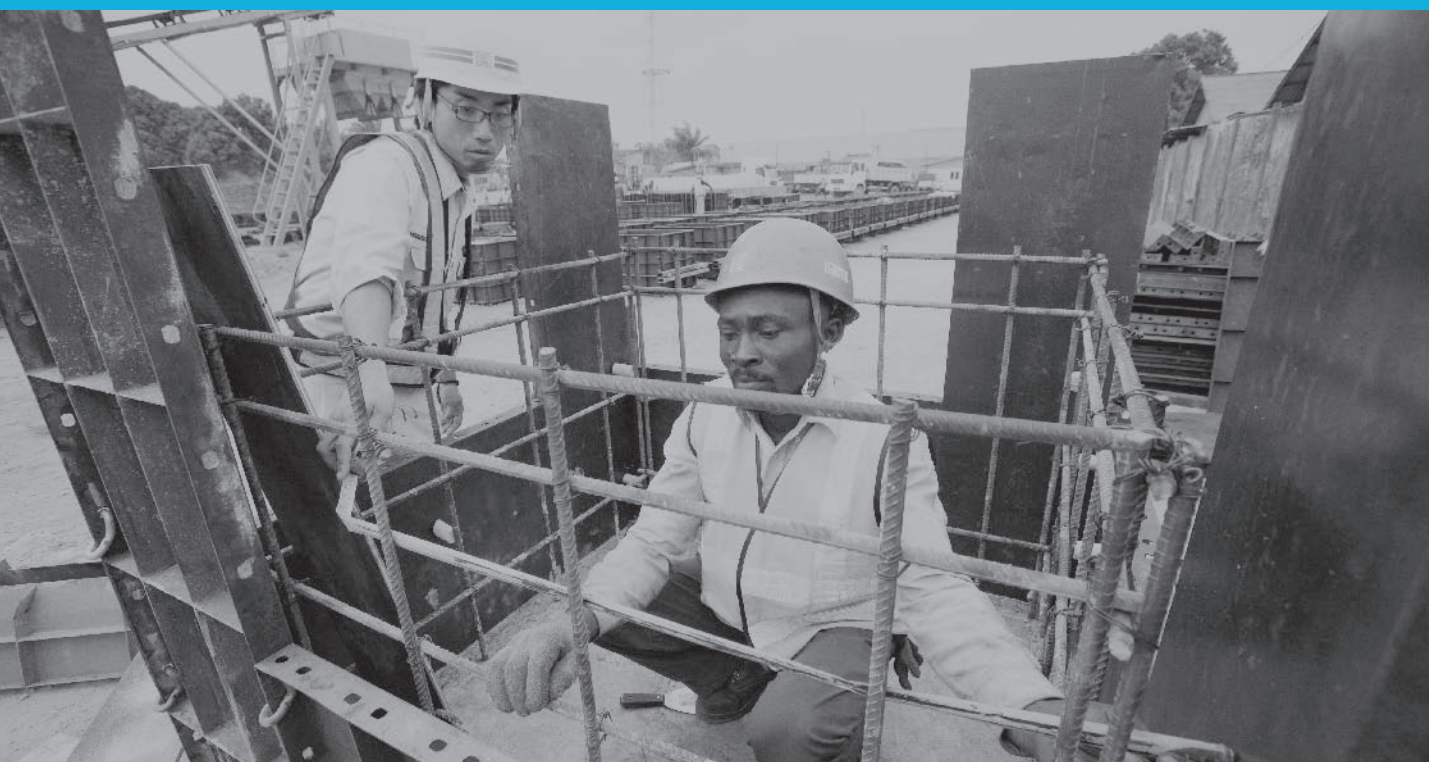
Japanese engineer and local staff working to improve and widen a traffic-congested main road in the Democratic Republic of the Congo (Photo: Shinichi Kuno / JICA)
