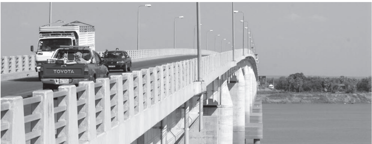
"Kizuna Bridge" in Cambodia (Photo: Kenshiro Imamura / JICA)
