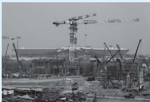
The second passenger terminal that is under construction. Behind it, the first passenger terminal that is used currently. (Photo: JICA)
