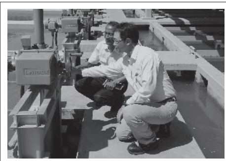
Confirmation is made about the valve update plan with the manager in charge of water purification at the Phum Prek Water Treatment Plant in Phnom Penh. (Photo: Takayuki Kawasaki)
