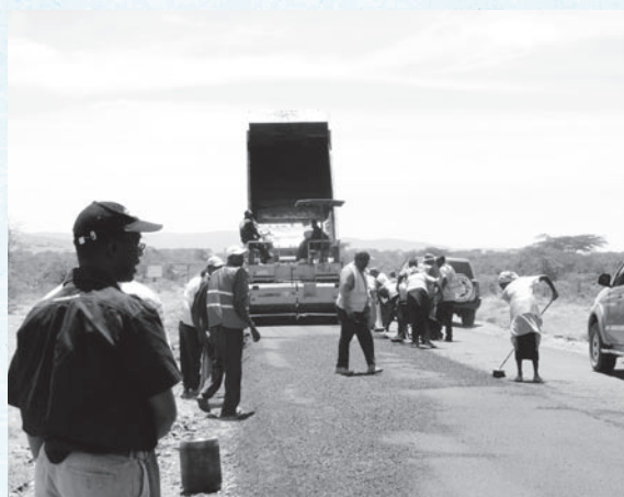
Pavement resurfacing work takes place along a road through savanna. (Photo: Motohiko Nishibayashi)
