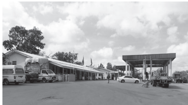
One Stop Border Post facility in Namanga on the Kenya-Tanzania border (Photo: JICA)
