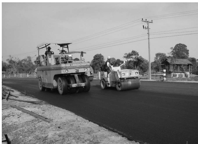
A project to improve roadway maintenance capabilities in Laos. Repairs were done in badly damaged areas. (Photo: JICA/International Development Center of Japan/Oriental Consultants)
