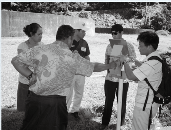
Checking the instruments that measure water volume in pipes at the Alaoa Treatment Plant (Photo: JICA)
