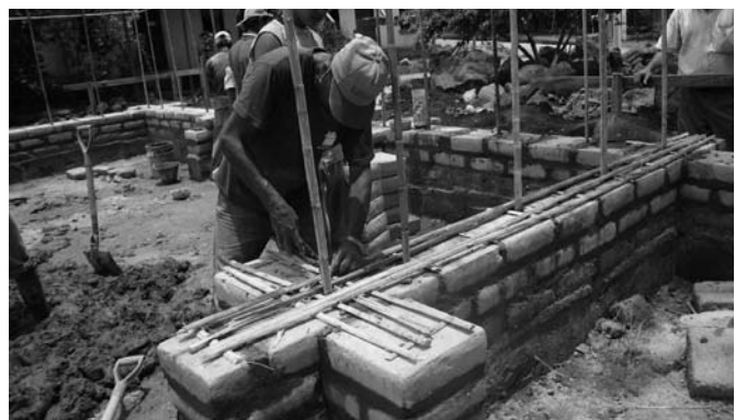
Construction of an earthquake-resistant model house with improved soil walls. Since 2003 Japan has cooperated with enhancing the earthquake resistance of houses and the proliferation of houses of high earthquake resistance in El Salvador which experienced two major earthquakes in 2001. (Photo: JICA).
