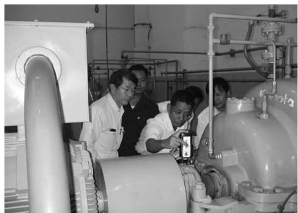
Japanese experts instruct the staff of the Phnom Penh Water Supply Authority on water supply facility maintenance. (Photo: Kitakyushu City Water and Sewer Bureau)
