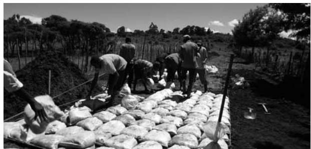
The use of CORE’s “Do-nou” construction method allows local residents to easily make repairs by themselves. (In Rift Valley Province, Kenya) (Photo: CORE)
