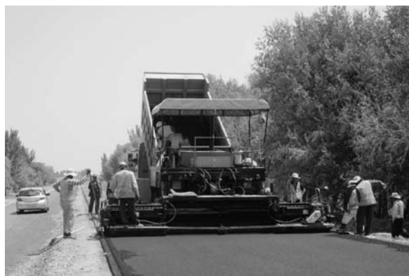
Construction work on the road from Kurgan Tyube to Dusti (Photo: JICA)
