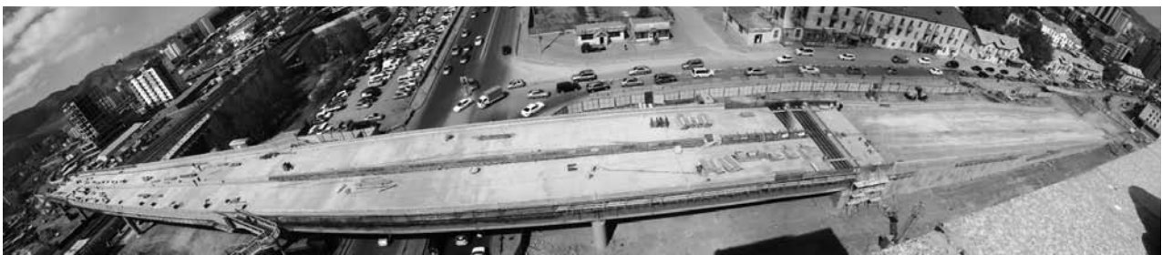
Sun Bridge, under-construction, straddling the railroad. (Photo: JFE Engineering)
