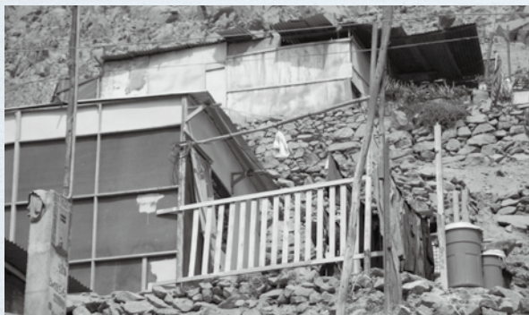
Homes on a steep slope. Plastic buckets (right) were used to carry water prior to the construction (Photo: Regina Torme)
