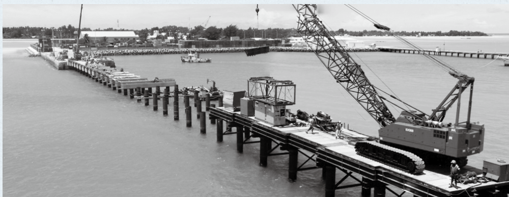
Full view of a bridge under construction with the container yard in the background (Photo: Masanori Anan)
