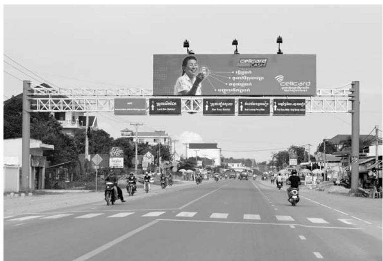
Construction is complete on the new, improved Cambodian National Route 1. (Photo: Koji Sato/JICA)
