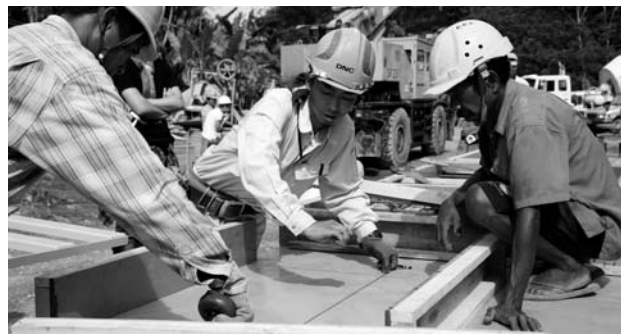
Japanese carpenters and basin residents work at a diversion weir upstream of the Bemos River in East Timor. (Photo: Shinichi Kuno/JICA)
