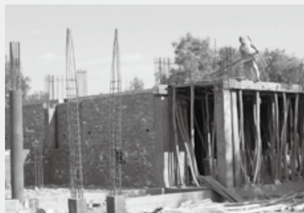
Emal Baba Higher Secondary School under construction. (Photo: UNDP)
