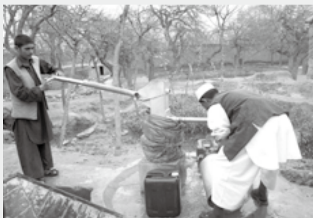
A well constructed in a DIAG development project. (Photo: UNDP)
