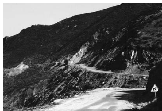
An unpaved road blocked by a landslide: Morocco
