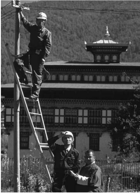
Communications network development to promote information technology in Bhutan (Project for Construction of the Domestic Telecommunication Network in the Western Region: Bhutan) (Photo: JICA)
