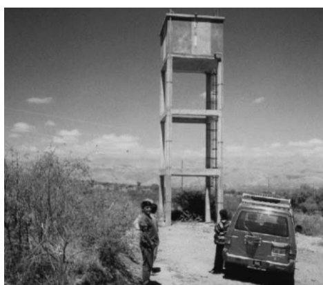
Water tower build by grant aid from Japan (Phase II Project for Groundwater Development in Rural Area in Bolivia)
