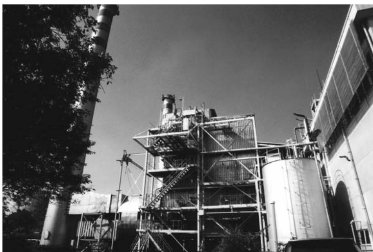
Tanjung Priok Gas Fired Power Plant in Indonesia
