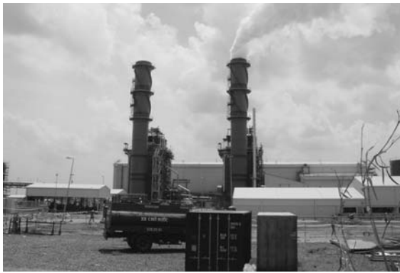
Phu My Thermal Power Plant in Vietnam (Photo: JBIC)
