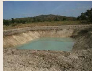
Building of additional agricultural ponds
