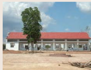
Renovation of elementary school buildings
