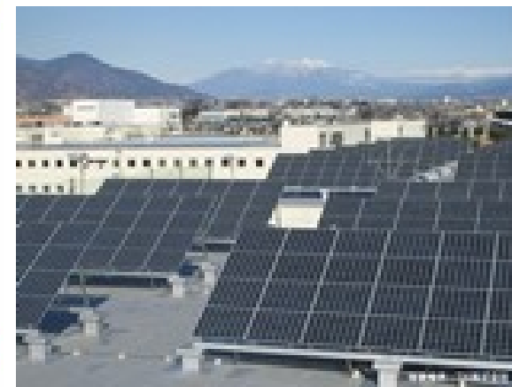
Large-scale solar panel installation on plant roof
