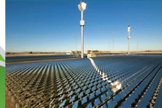
Concentrating solar Thermal power plant
