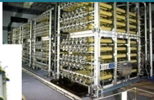
Water treatment unit
