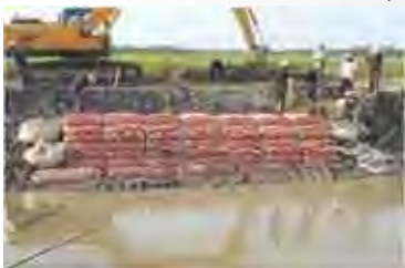
③ Installation of LS-100 with sand
