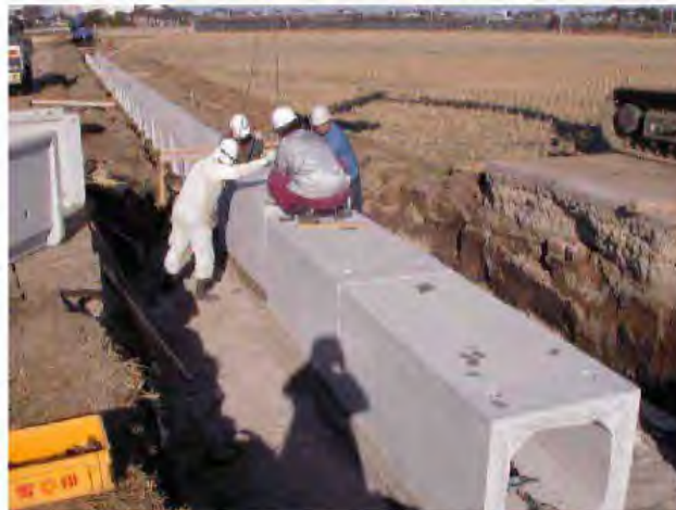
Installation of the box culvert /settlement of five months after is 3 mm-5mm only There is no subsequent subsidence as of now.
