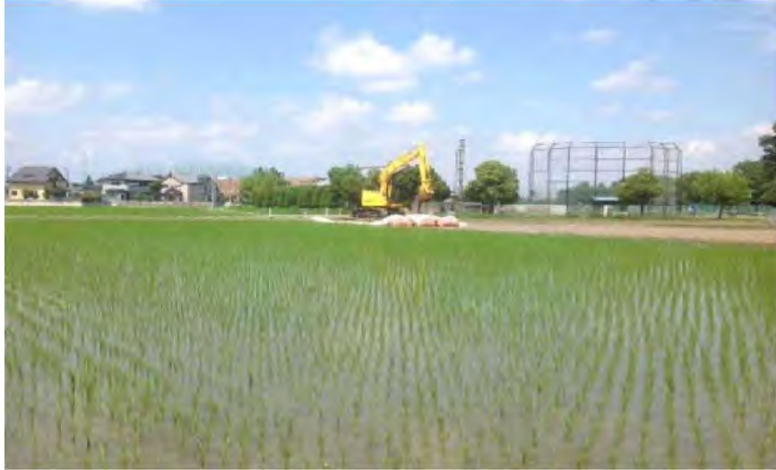
Temporary road at the very soft ground of rice field
