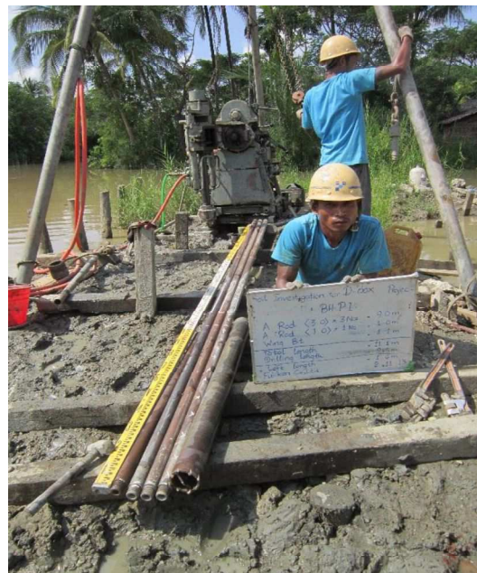
Drilling & Left Length (B)
