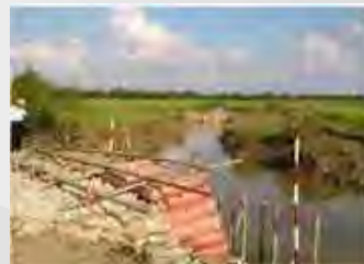
④ Completion of Slope by LS-100
