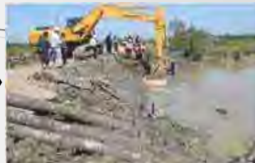
② Basement of slope LS150
