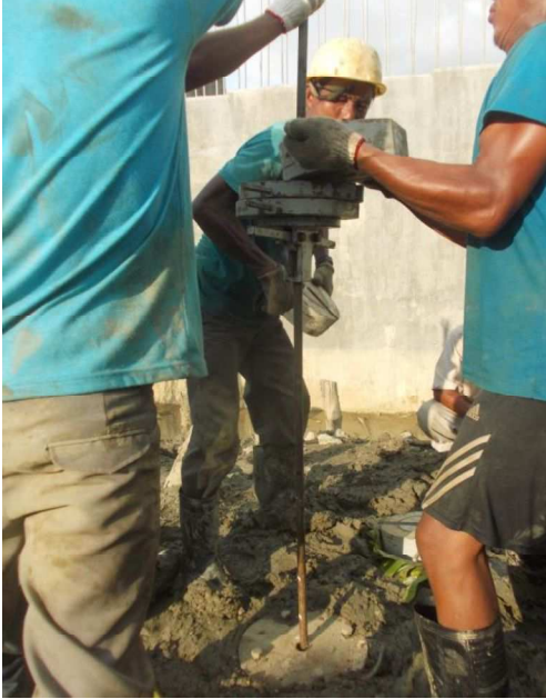
Before commencement of test work
