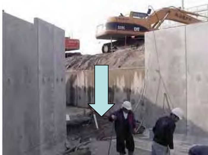
L type of Retaining wall with width 4m,height5m
