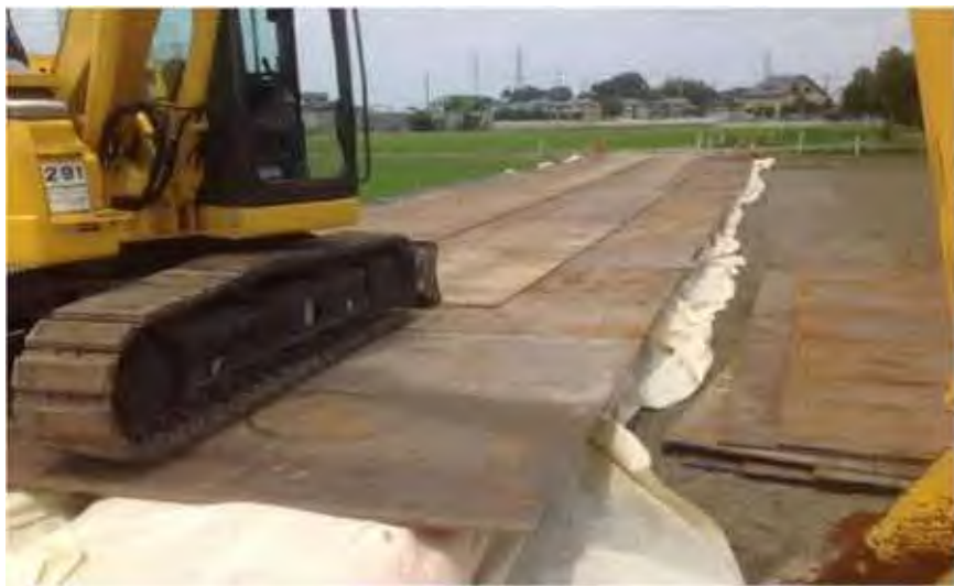
Steel sheet plates were installed on D. BOX in order to prevent damage from a heavy equipment
