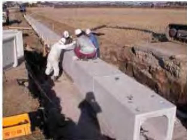
Installation of the culvert box /settlement of five months after is 3 mm-5mm only There is no subsequent subsidence as of now.
