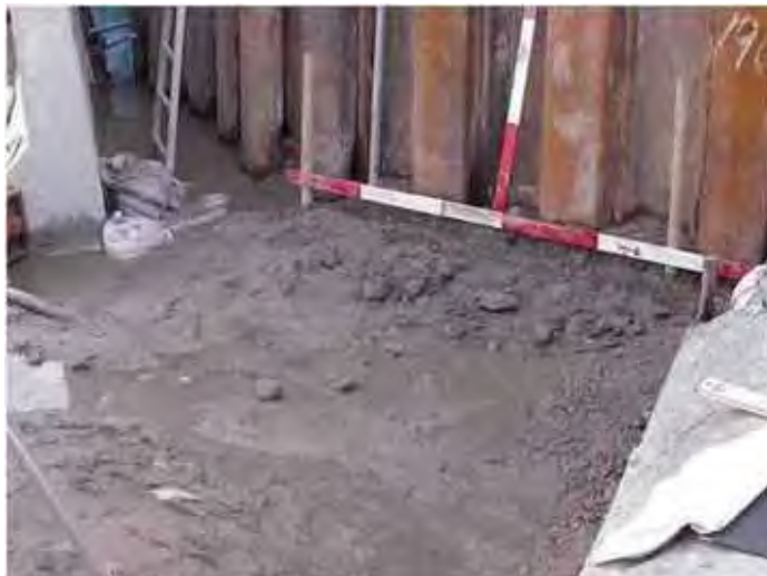
Before excavation ,Water is oozed out.
