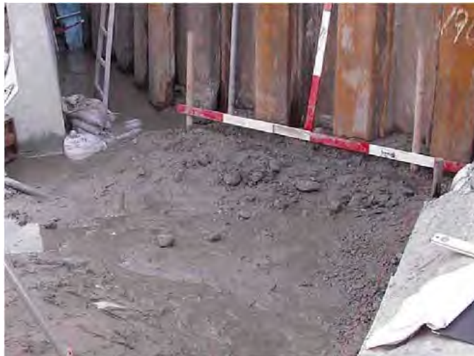
Before excavation ,Water is oozed out.
