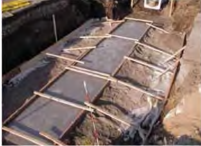
Base Concrete (casted a day after installed D-Box)
