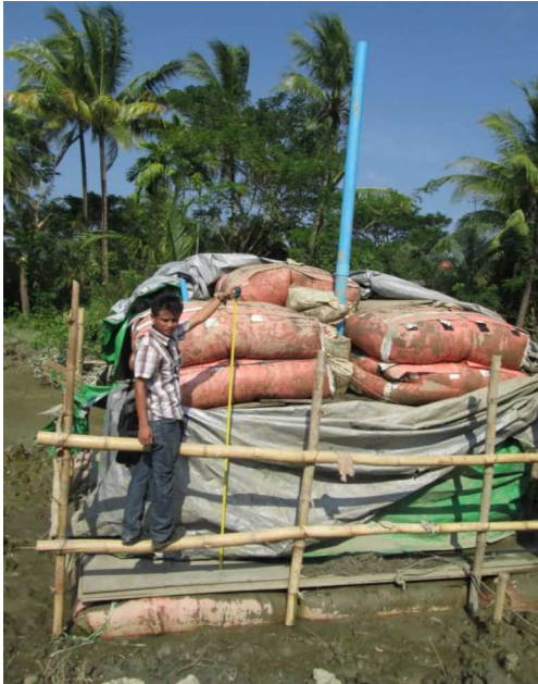
Before commencement of test work
