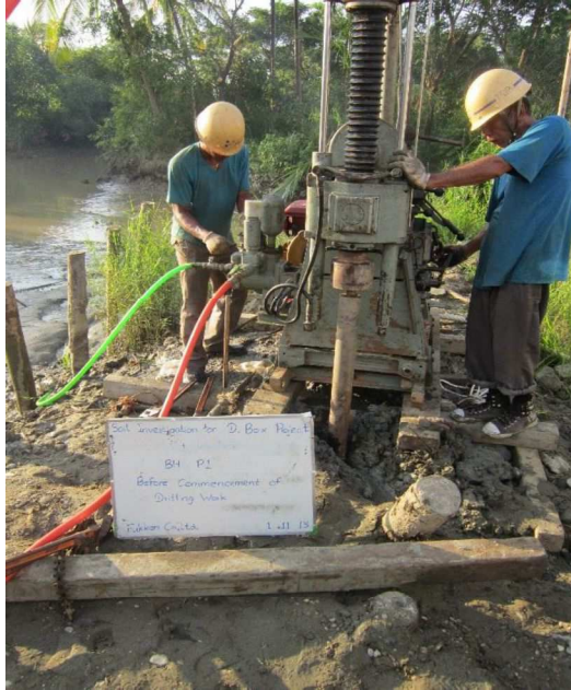
Before commencement of drilling work
