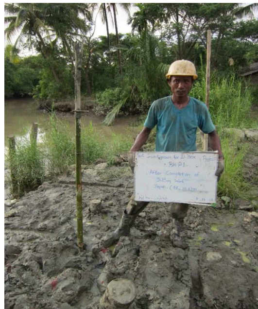
After completion of drilling work
