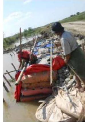
D·BOX is covered with blue sheet in order to protect from ultraviolet rays.
