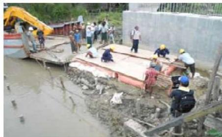
③ Back-hoe was able to land on the soft clay at Kyon Sein bridge using D-BOX
