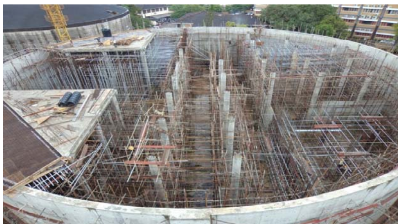
Construction of Ground Reservoir progress up to end of November 2013
