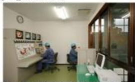
Central monitoring room
