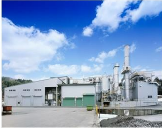
Incineration plant (Processing capacity 88.8ton/day)
