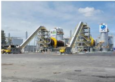
Ishinomaki city Facility for JFE ENGINEERING 300 ton rotary kiln × 2
