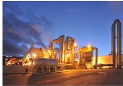
Kesenuma city 200 ton rotary kiln × 2
