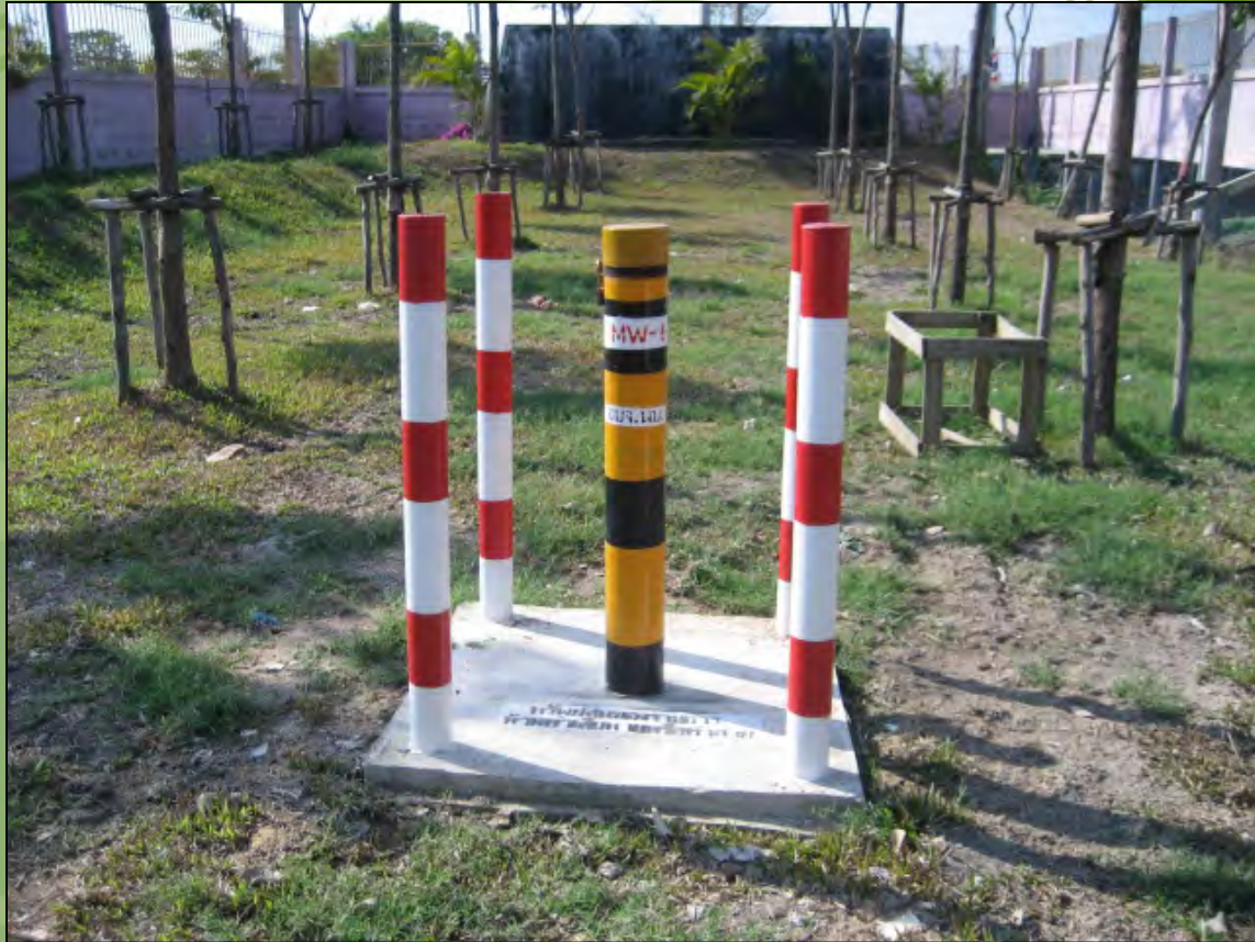
Underground water monitoring well
