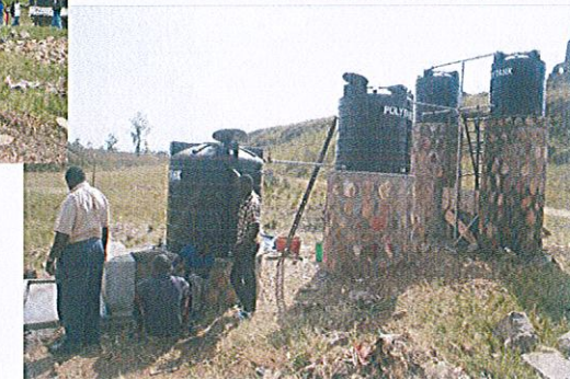
Completed water treatment plant
